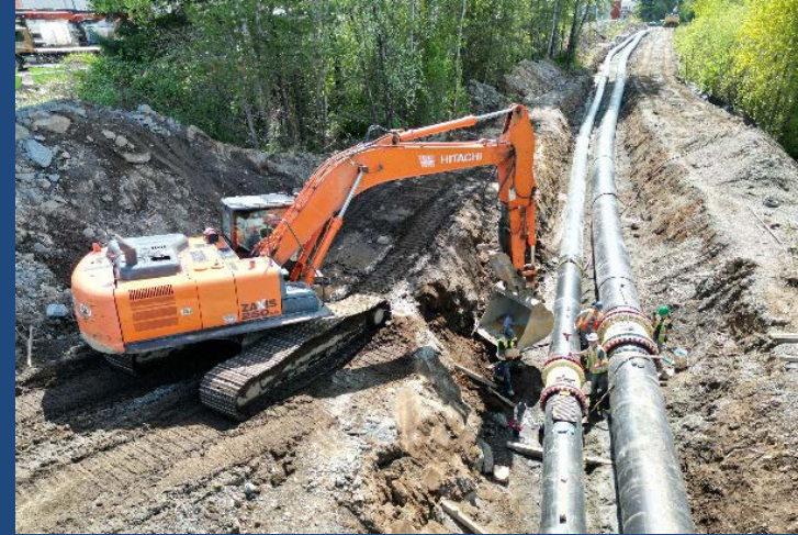
Midtown Water Supply Project
