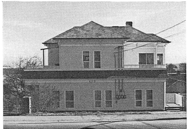
Figure 31 This conversion has successfully utilized flat roof areas as private outdoor open space without adversely affecting the character of the building.
