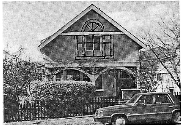
Figure 47 This sketch illustrates a way to enhance the appearance of this lovely older home by using an appropriate replacement window.
