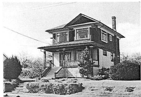
Figure 48 An example of the traditional layering of materials, expressing the base, main floor, and the cap.
