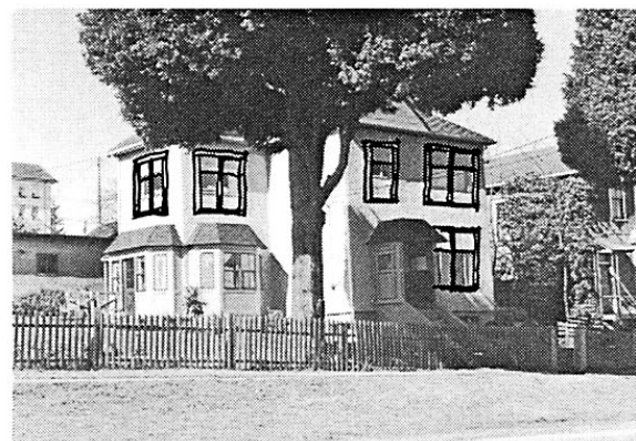
Figure 42 Using new windows with traditional proportions results in an attractive composition.
