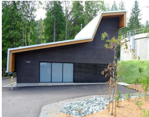
The Energy Recovery Facility and the Reservoir #1 drinking water storage tank
