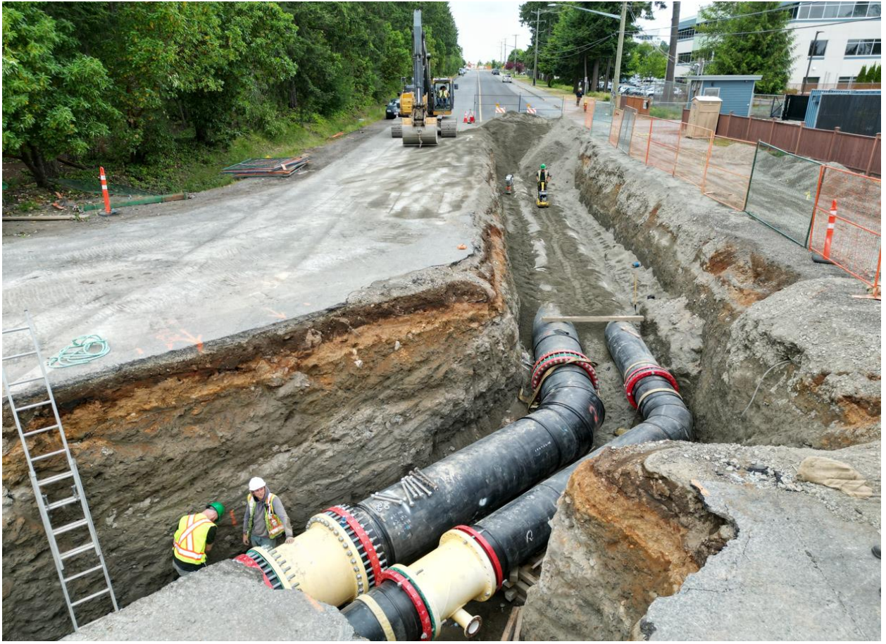
Construction of the new twin pipelines in Labieux Road, June 2023
